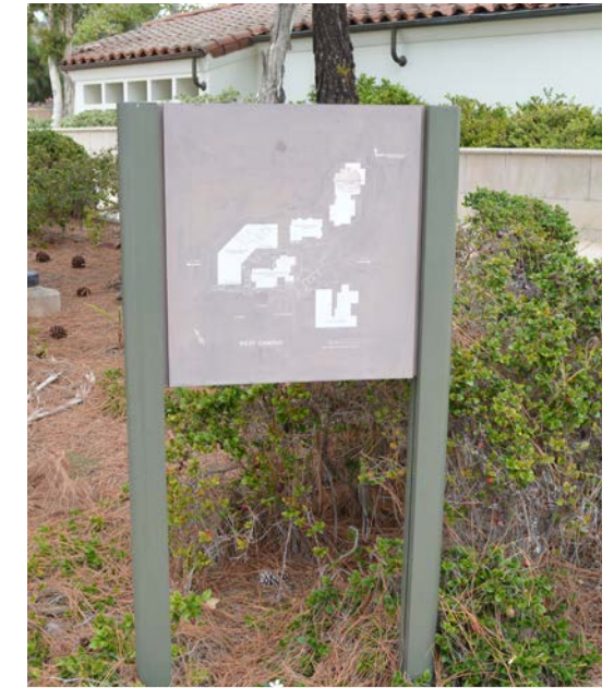
Existing signage has legibility issues and is in disrepair
