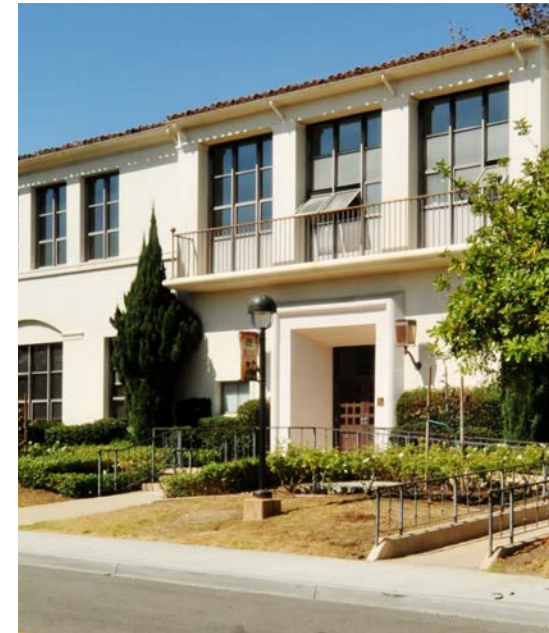
The Administration Building features the terracotta tile, ironwork, and white stucco of the Santa Barbara style.
