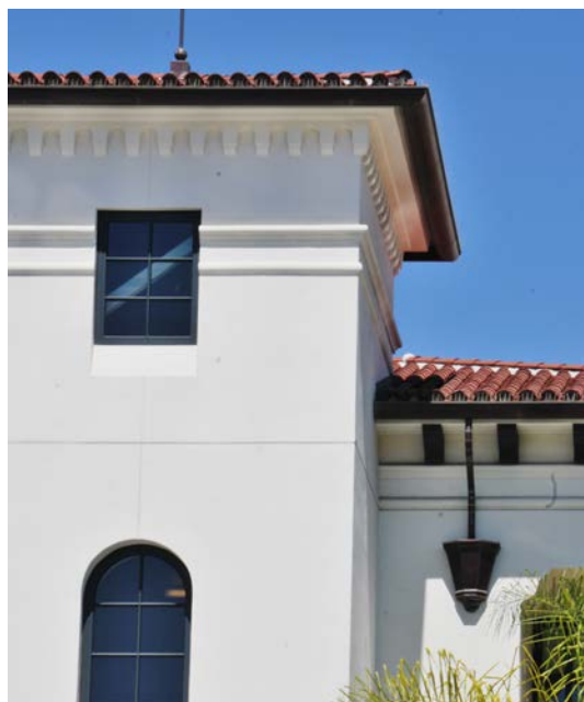
An otherwise plain facade is articulated through the use of trim, cornice bracketing, and recessed windows with varying shapes.
