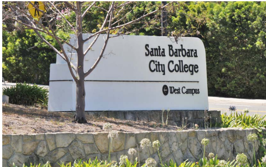
West entry at the Main Campus is identified, however the sign is located away from the roadway and not visible from a distance.
