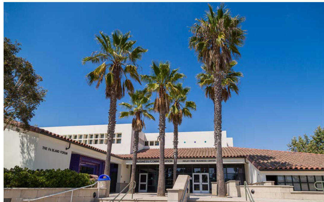
The Business Communications Building uses multiple types of window and opening types to break up the long facade surfaces and to achieve a more human scale. The ramps are incorporated into the entry.
