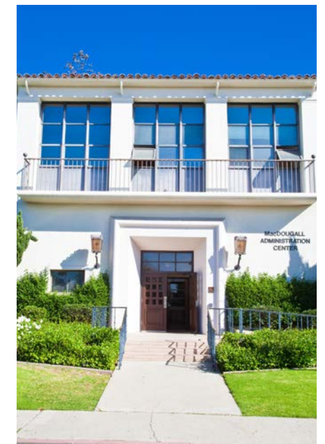
The Administration building has a clearly articulated entrance and integrated ramp access.
