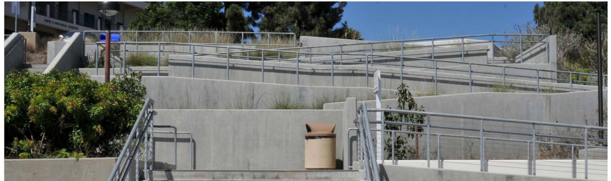
Minimize ramps requiring handrails by designing paths of travel under 5% where possible.
