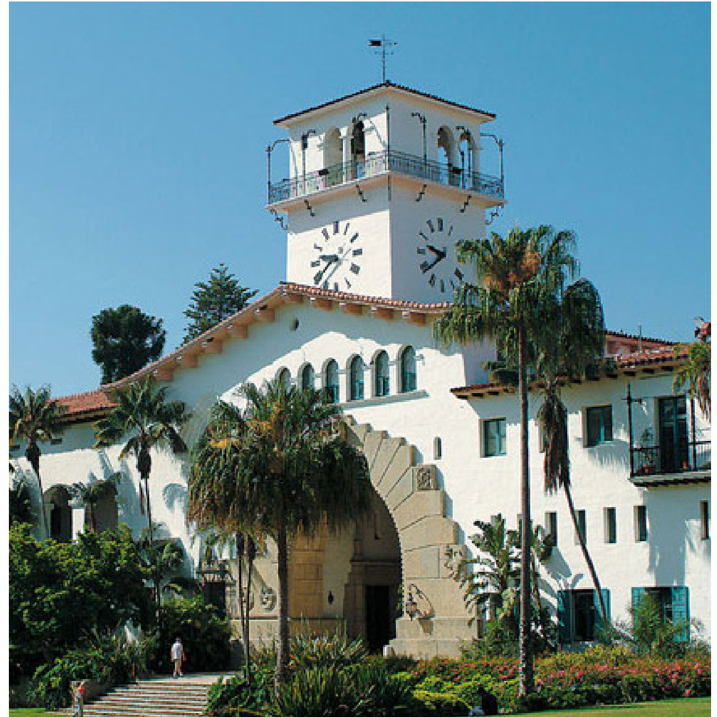
Completed in 1929 and designed by William Mooser, the Santa Barbara County Courthouse exemplifies the 'Santa Barbara Style' of architecture with its decorative ironwork, smooth plaster walls, clay tile roofs, and arched openings.
