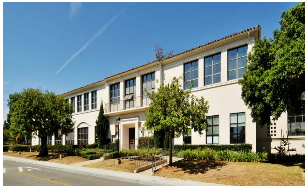
The Administration Building on the Main Campus would be an intimidating building were the massing not broken up into distinct volumes by stepping portions in and out and by using large windows with limited but effective variations in size and shape.
