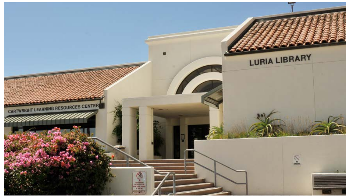
The Learning Resources Center on the Main Campus uses an arched opening and covered portico to clearly indicate the main building entrance.
