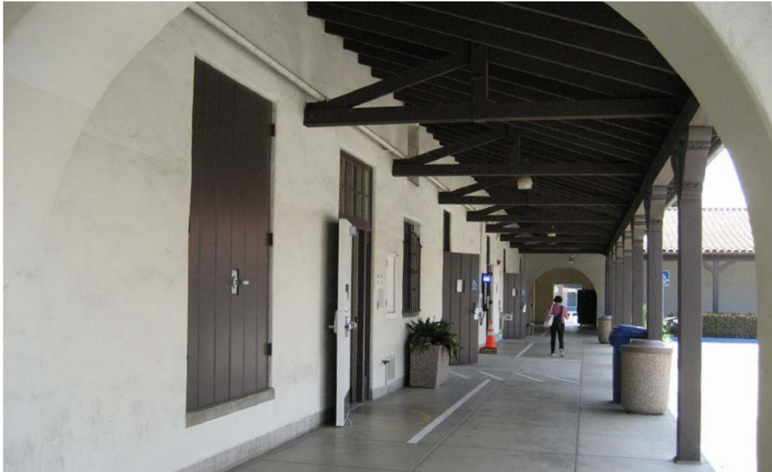
The Spanish Colonial Revival style featuring arched openings and arcades with exposed timber is consistent across the Schott Campus.
