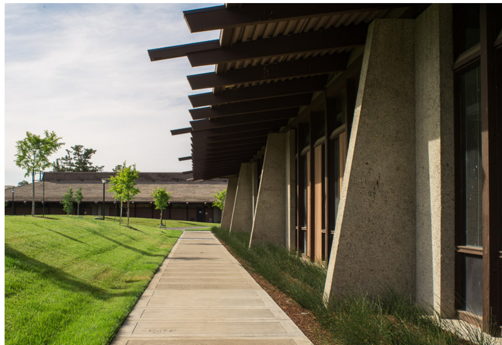
Grading of turf directs stormwater into swales and minimizes unwanted pooling.
