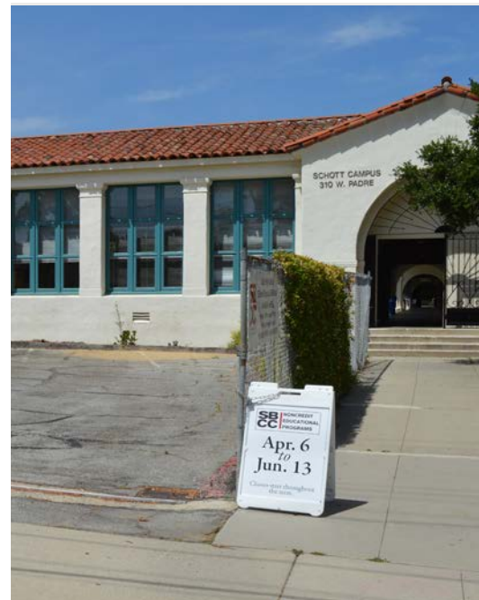
The entrance to the Schott Campus building and parking lot
