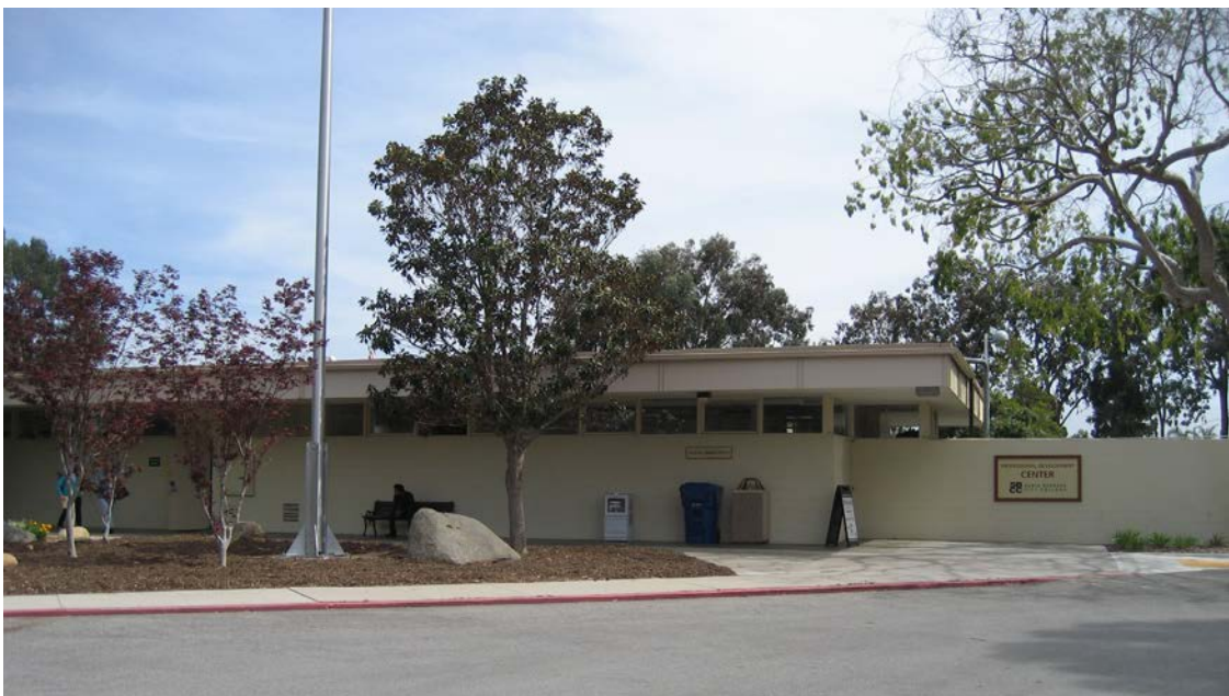
The original buildings featured clerestory windows to admit light and ventilation without distracting students with views.
