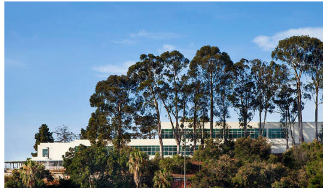
The Humanities Building is designed to harmonize with the ground plane and topography so as not to be obtrusive, in spite of being more than one story high.
