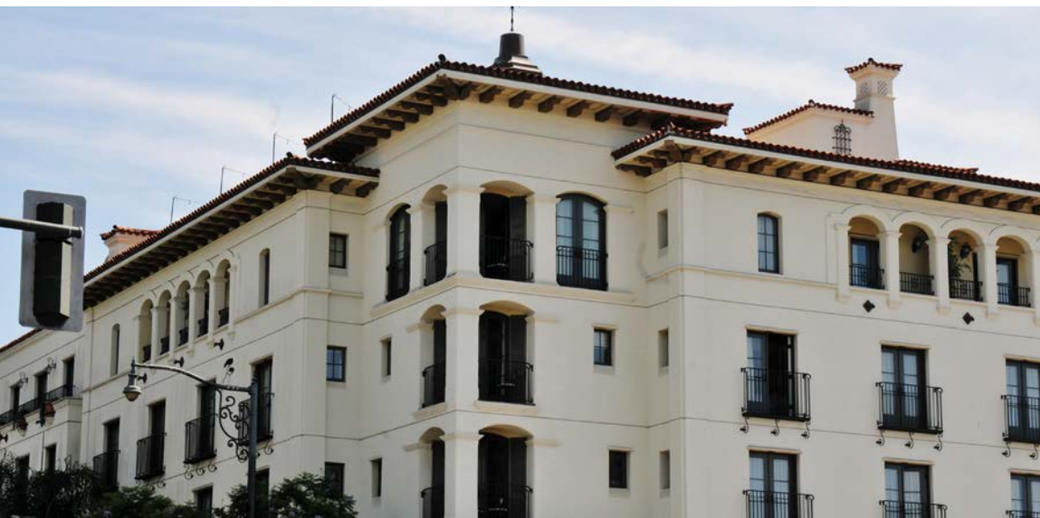
This large downtown building is broken down into a more accessible scale by recessing the corner into towers, varying the cornice and roof line heights, and providing deeply recessed apertures.
