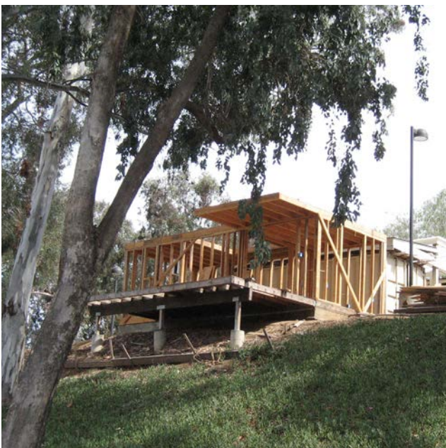
Construction Academy projects at Wake Campus
