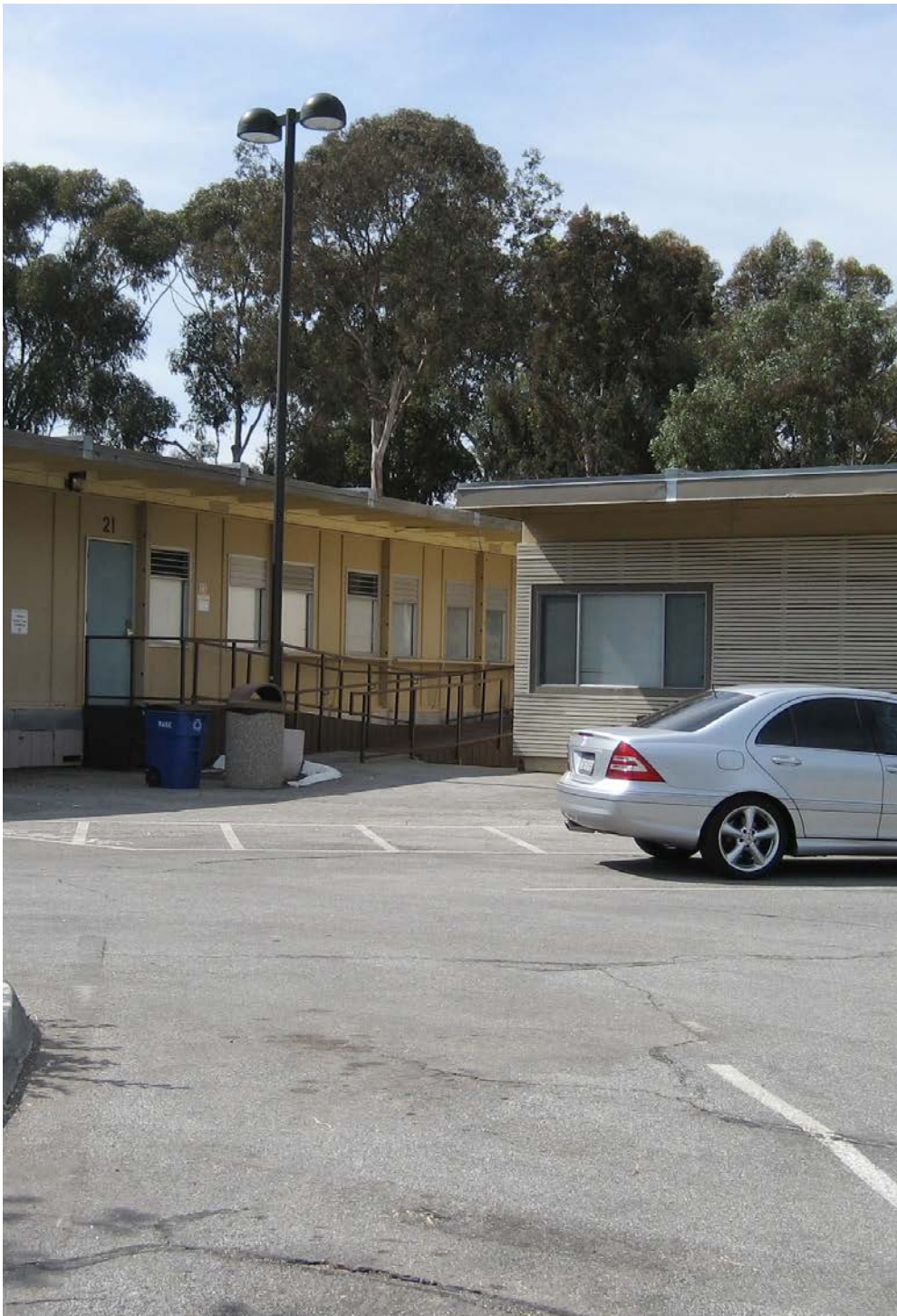
Modular buildings and unpermitted additions at Wake Campus
