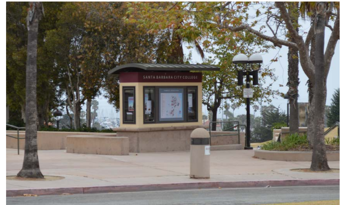
Within the very inconsistent current signage, the newer information kiosks are functional and are well constructed and in good condition
