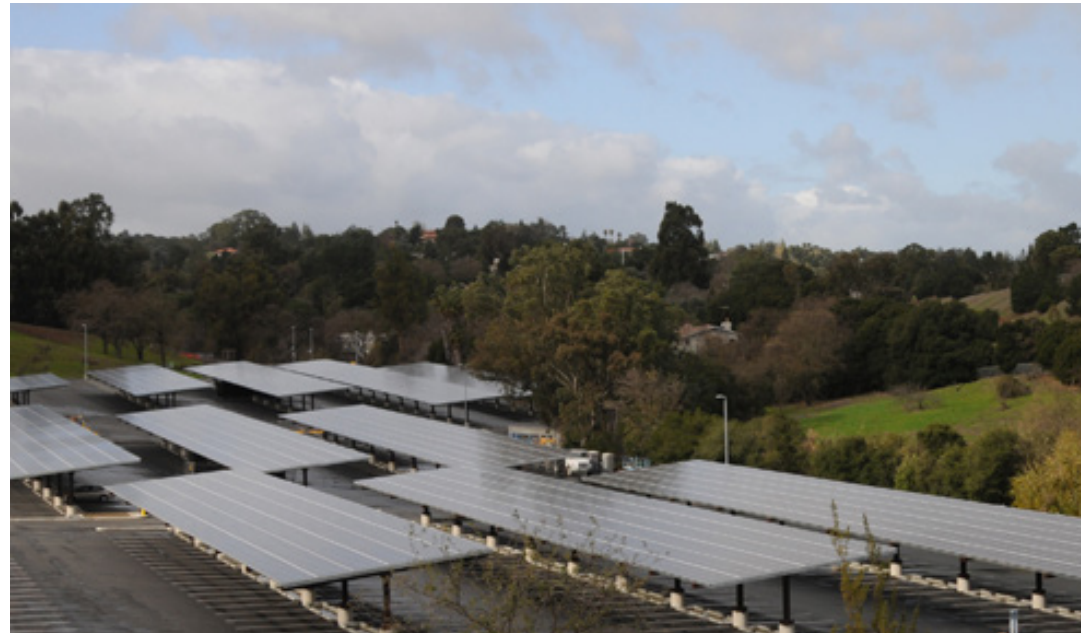
Solar panels can contribute to the overall identity of the college.
