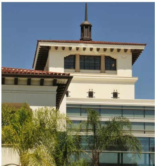
The curtain wall glazing in this hospital reflect varying depths in the facade between the glazing, mullions, and wall surface.
