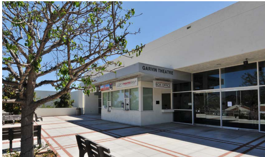
Providing shading at large glazed openings helps minimize air conditioning costs, as in the Garvin Theater.
