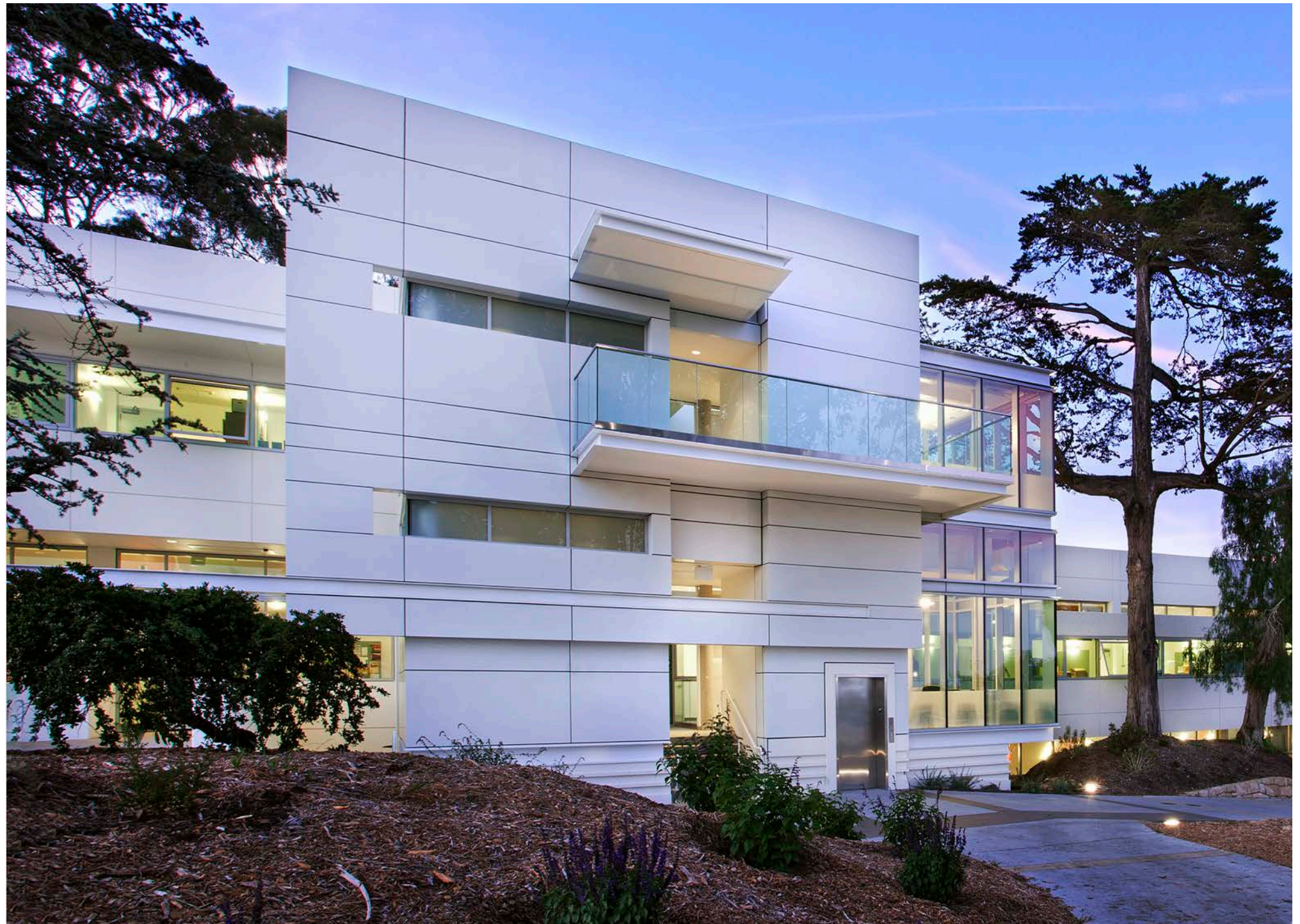
The Humanities Building is in a modern style, but has a white stucco finish and a close relationship to the ground plane emphasized by the horizontal joint lines.
