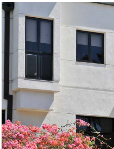
The cantilevered bay of this window create a visual break in an otherwise long flat facade.
