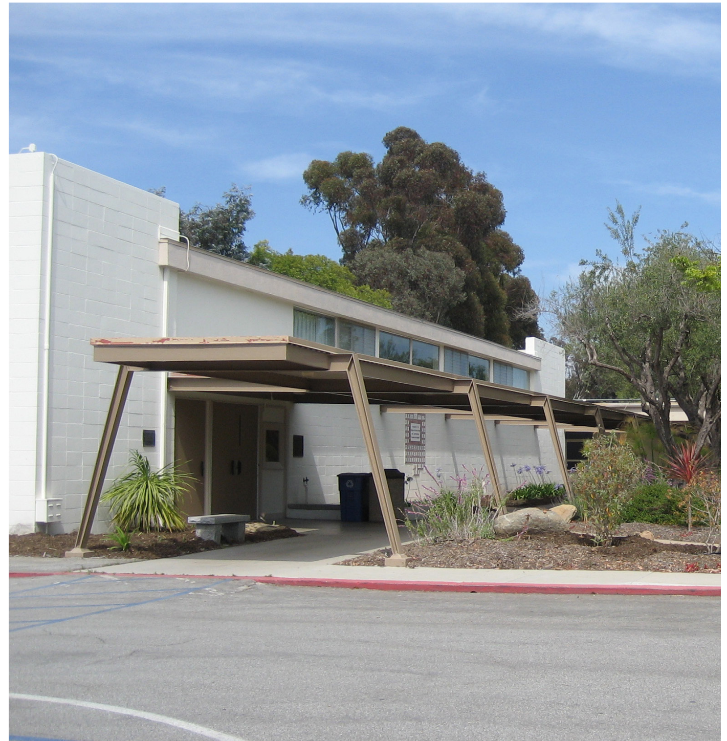
Visitors to the Wake Campus are greeted at the main entrance by a Modernist concrete masonry unit building and a painted steel breezeway with canted I-beam columns.
