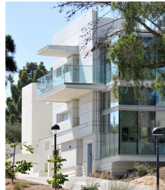
The Humanities Building's uses white stucco in a more modern pattern of horizontal, linear pattern of joints.
