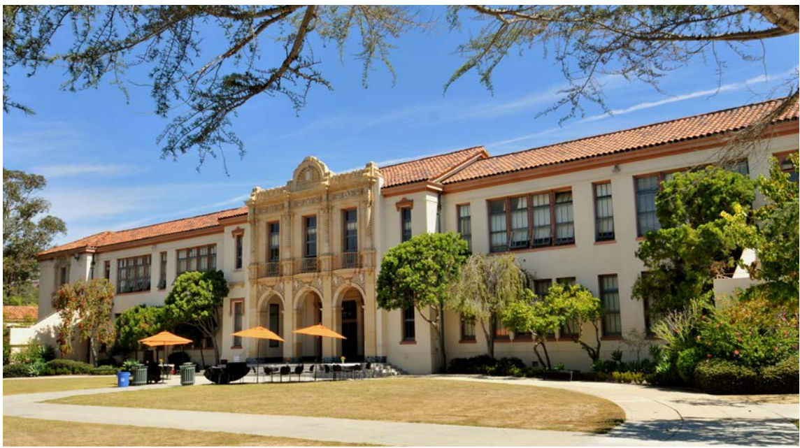
Similar to the Administration Building, this long building is broken into a more human scale by slight shifts in the roof lines, facade articulations, and window groupings.
