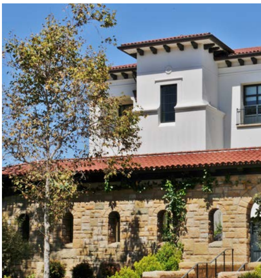
This Santa Barbara building broke up its massing by setting back the upper floors and changing the facade materials.
