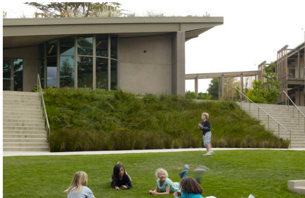
A hillside smoothly graded to work with the rise of the intersecting stairs and planted for slope stabilization
