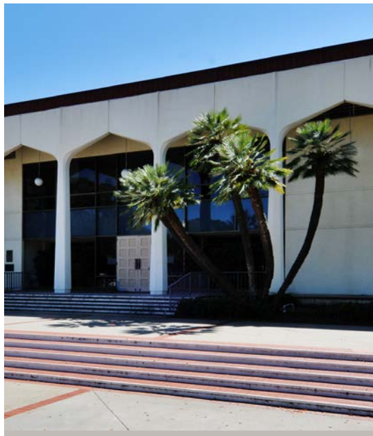
The Student Services Building references classical architecture in its double height arcade but uses Santa Barbara materiality.
