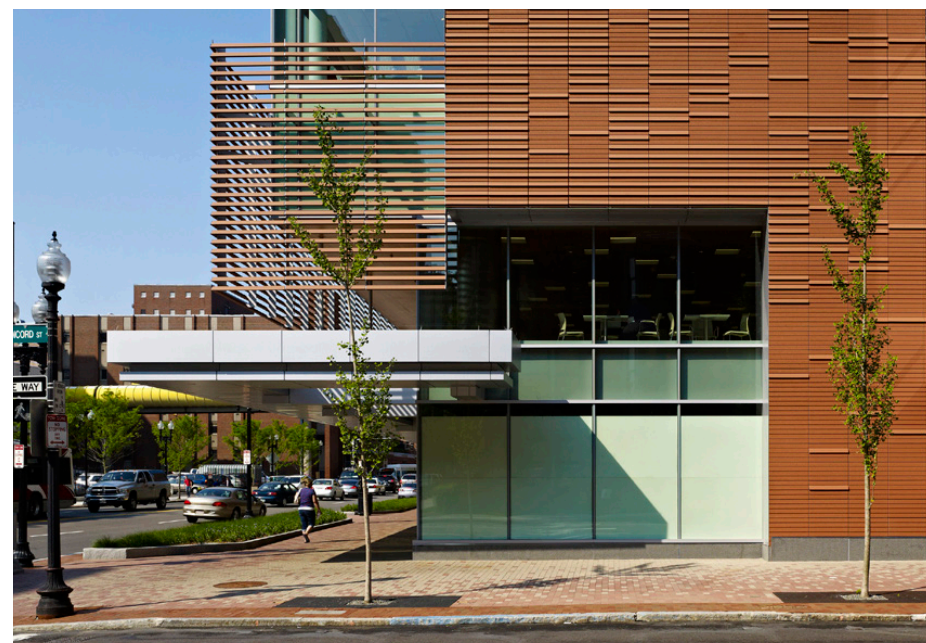
Designers could use materials found on the SBCC campus in new ways. In this building, terracotta baguettes are used as a screening rather than roofing material. (Photo by Jeffrey Totaro)
