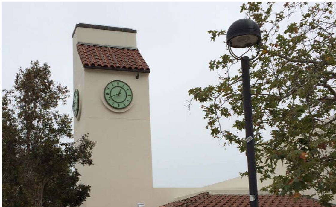
Green accent color used at the clock tower on the Main Campus
