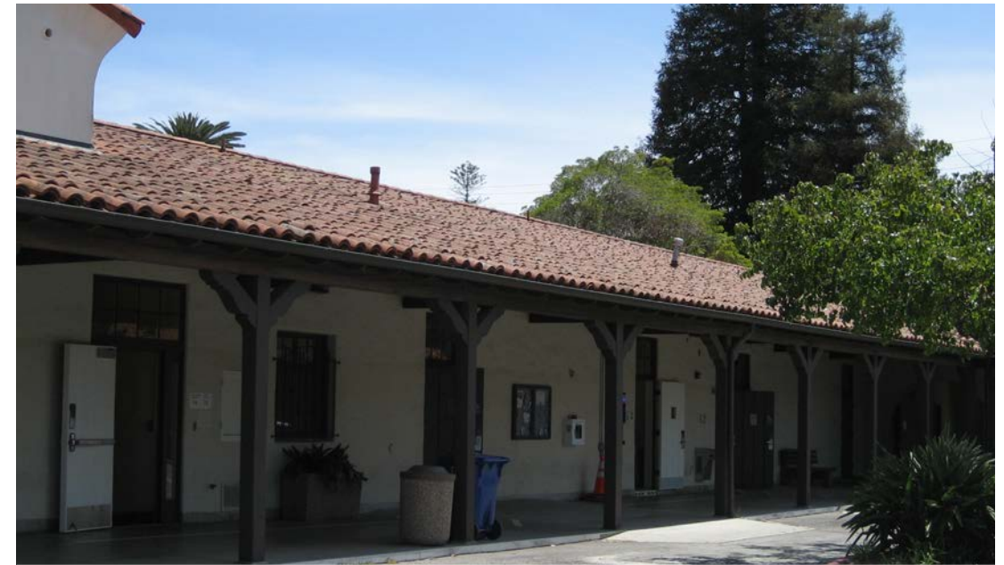
This pedestrian scale arcade at Schott Campus is a common feature of the Spanish Colonial Revival and Santa Barbara styles. However, the arcade has an abrupt transition to the parking lot.
