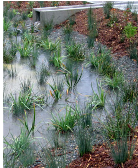
A swale inundated in a storm event provides an opportunity for teaching.
