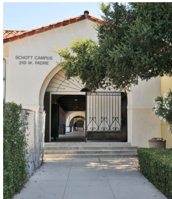
Main entrance at Schott Campus
