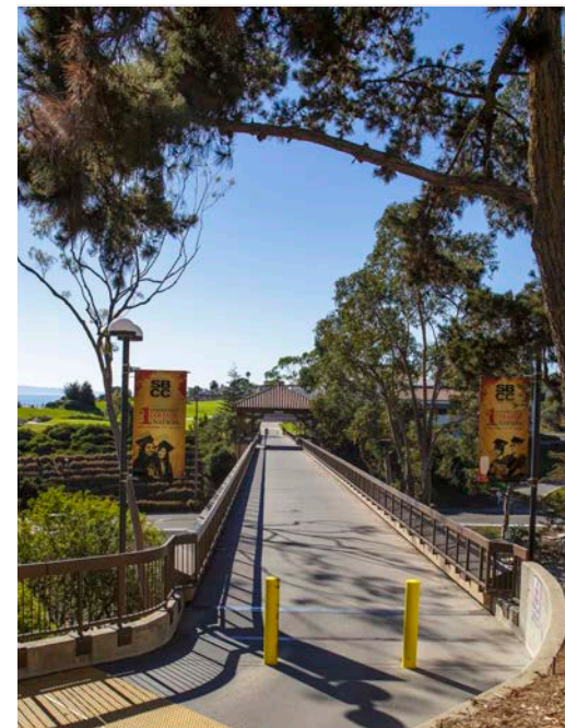
Loma Alta bridge connecting the east and west sides of the Main Campus.
