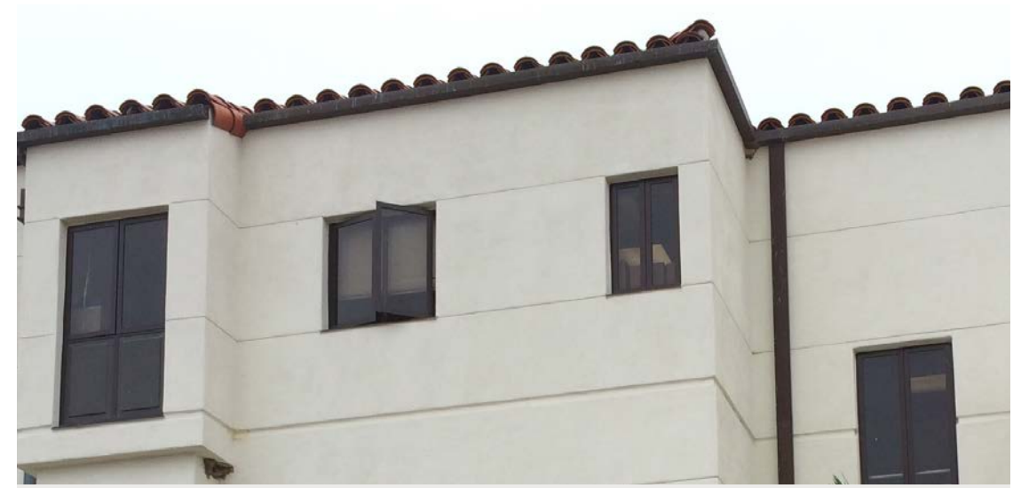
Dark bronze metal finish on window frames, downspouts, trim
