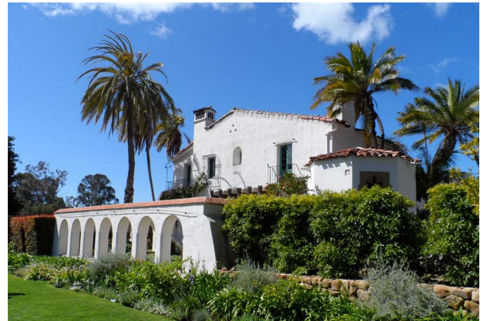
An arcaded exterior walkway extends into the landscape and defines space at the Casa del Herrero.
